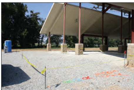
The Farmers' Market pavilion before the deck was finished.
